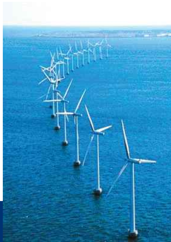
Offshore wind farm.
